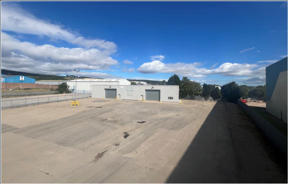
External of Building 2
