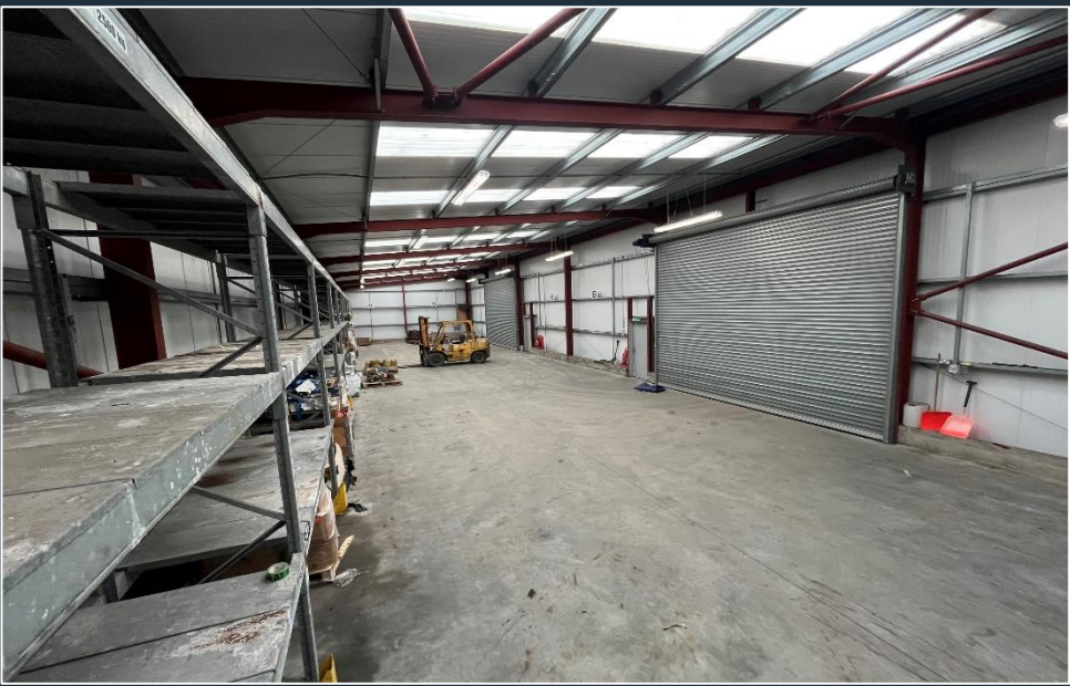
Internal of Building 2 *Nearing completion of refurbishment programme.
